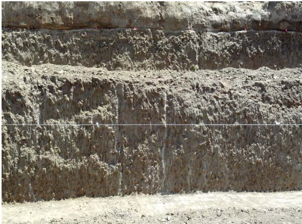
Photo 18 – Discontinuous Fractures – Station 0+90
