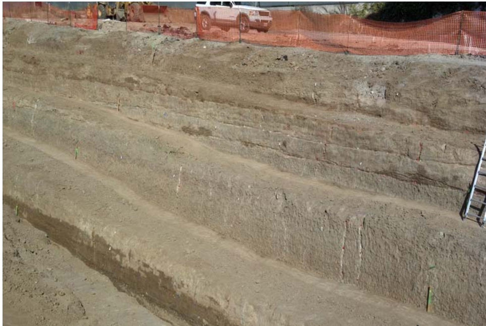
Photo 8 – Continuity of Geologic Units-Central Portion of Trench
