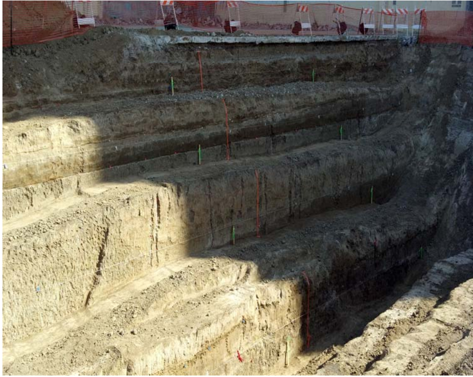
Photo 13 – Soil Profile 1 – Station 0+46
