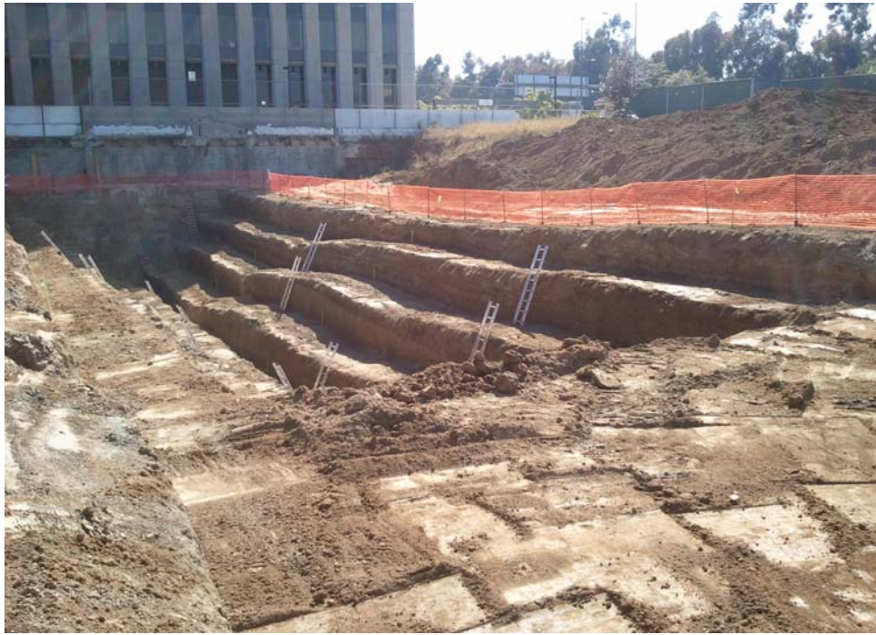
Photo 1 – Trench Excavation Looking West
