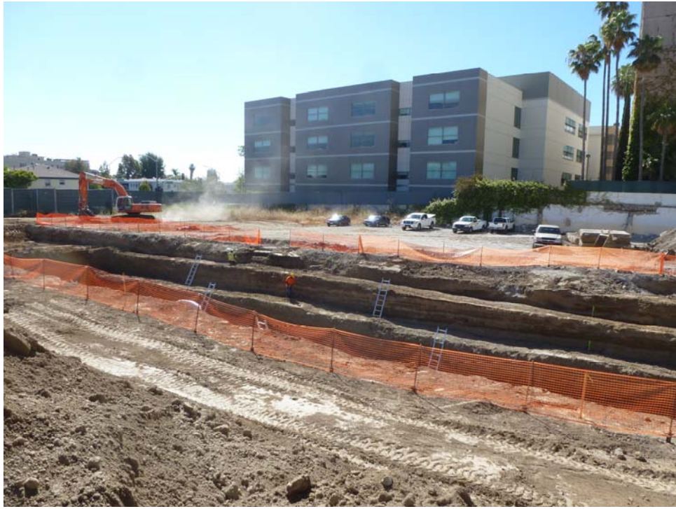
Photo 5 – Trench Excavation Looking East-Southeast
