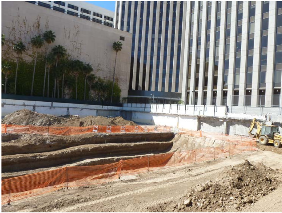
Photo 3 – Trench Excavation Looking South
