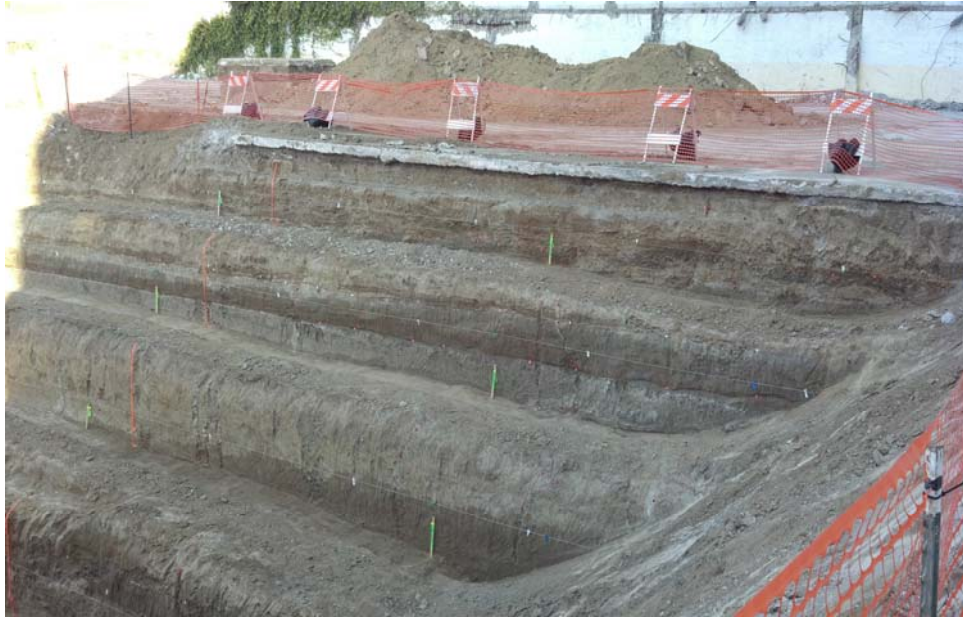
Photo 7 – Continuity of Geologic Units-Western Portion of Trench
