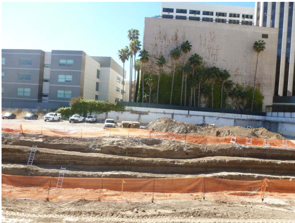
Photo 4 – Trench Excavation Looking Southeast
