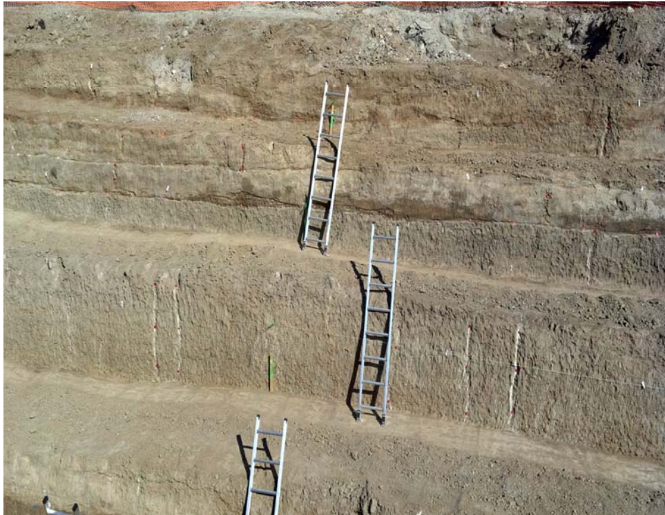
Photo 15 – Discontinuous Fractures – Station 1+00
