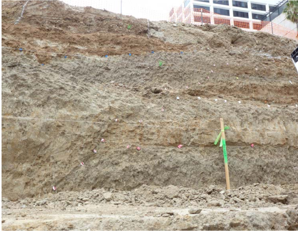
Photo 11 – Paleochannel Boundary-Southeast Trench Wall
