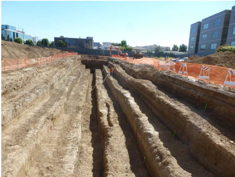
Photo 6 – Trench Excavation Looking East
